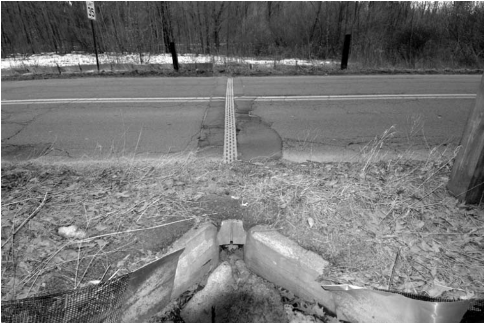
Figure 6-6. Salamanders use this tunnel to cross under a road during their annual migration to breeding ponds. Note the fencing and concrete “funnel” in the foreground of the photo, which guide salamanders toward the underpass and prevent them from accessing the road surface.
