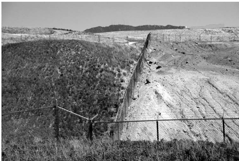
Figure 9-6. Reclamation efforts in Butte have transformed old mine tailings sites from bare, metal-laden earth, as seen on the right, to sites covered with native grasses, as on the left.
