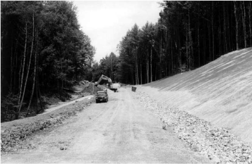
Figure 10-5. Requirements for wide roads, shallow grades, and long sight distances translate into the need to destroy and regrade large amounts of native habitat.
