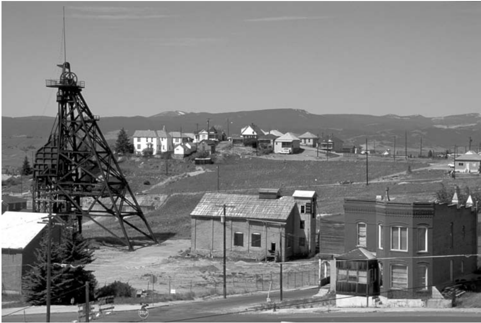
Figure 9-2. In Butte, Montana, copper mining has taken place for over a century. Here, a headframe, which stood over the top of a mine shaft, still stands in a Butte neighborhood.
